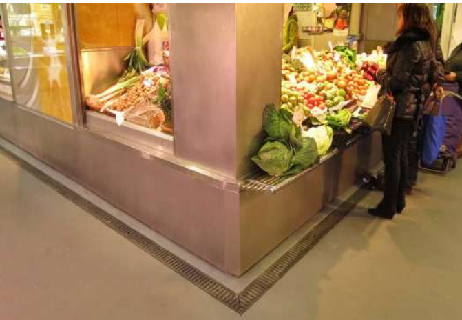
Drainage channels at the Ribera Market in Bilbao- North Spain. Courtesy: ULMA Architectural
