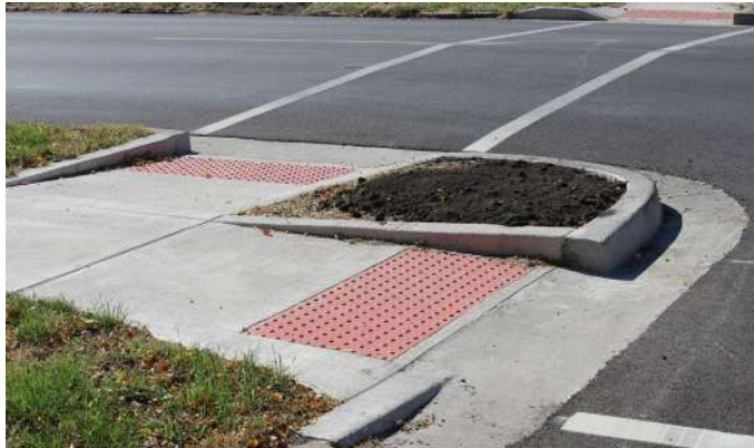
Kerb Ramps with tactile ground surface indicators, Illinois Photo Credit: Maurer-Stutz
